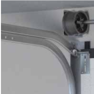
Ⓒ Double track sliding mechanism
