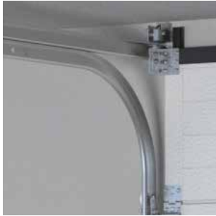
C Double track sliding mechanism
