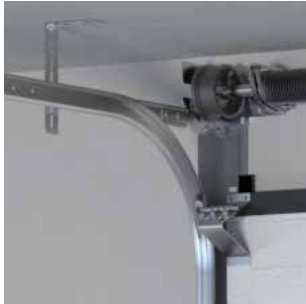
Ⓒ Single track sliding mechanism
